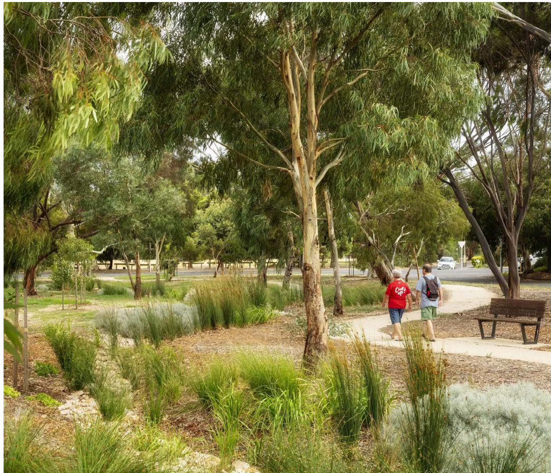
Vegetated detention basin
